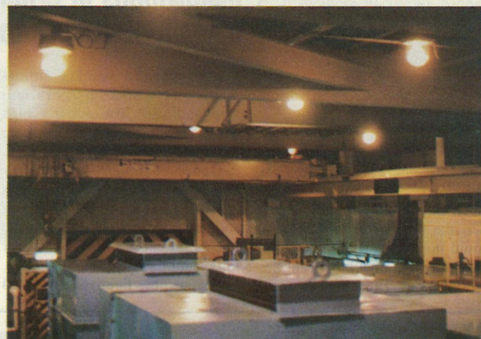
Effective lighting using high wattage Ex(d) luminaires — fourteen of these fittings replaced more than 200 fluorescent luminaires.
